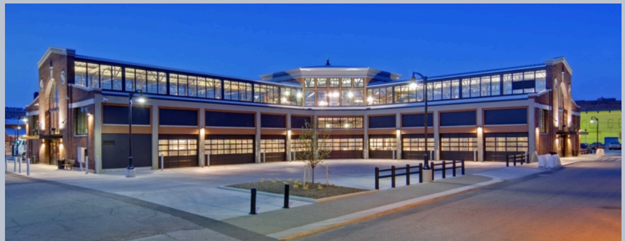
Eastern Market Shed 3 Renovation | Detroit, MI
