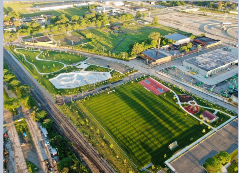
Riverside Park—Phase I & II | Detroit, MI
