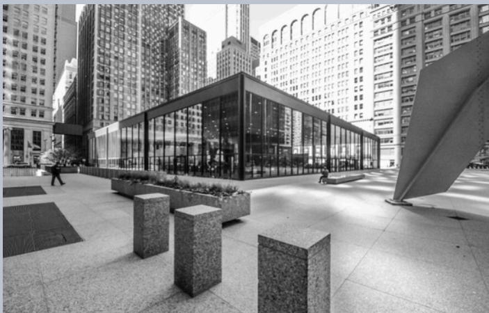
Loop Station, Chicago, IL
